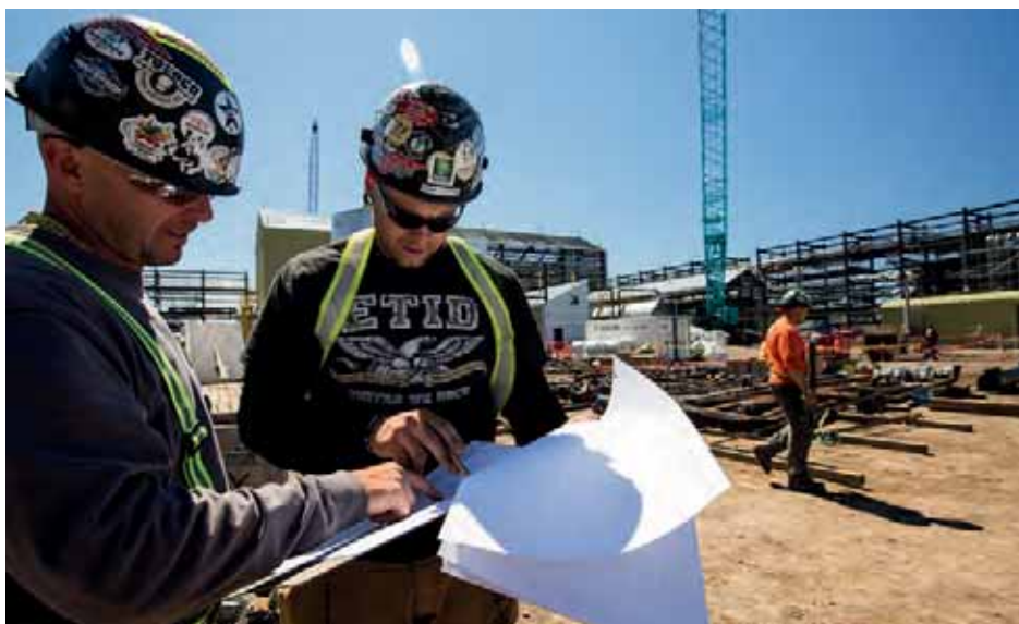
In partnership: workers (above) at the Sunrise project, Alberta; Susan Casey, safety advisor (middle), is part of a safety team that has promoted a strong safety culture onsite; and an onsite fire and rescue squad (far right) trains rigorously in order to stay prepared.
