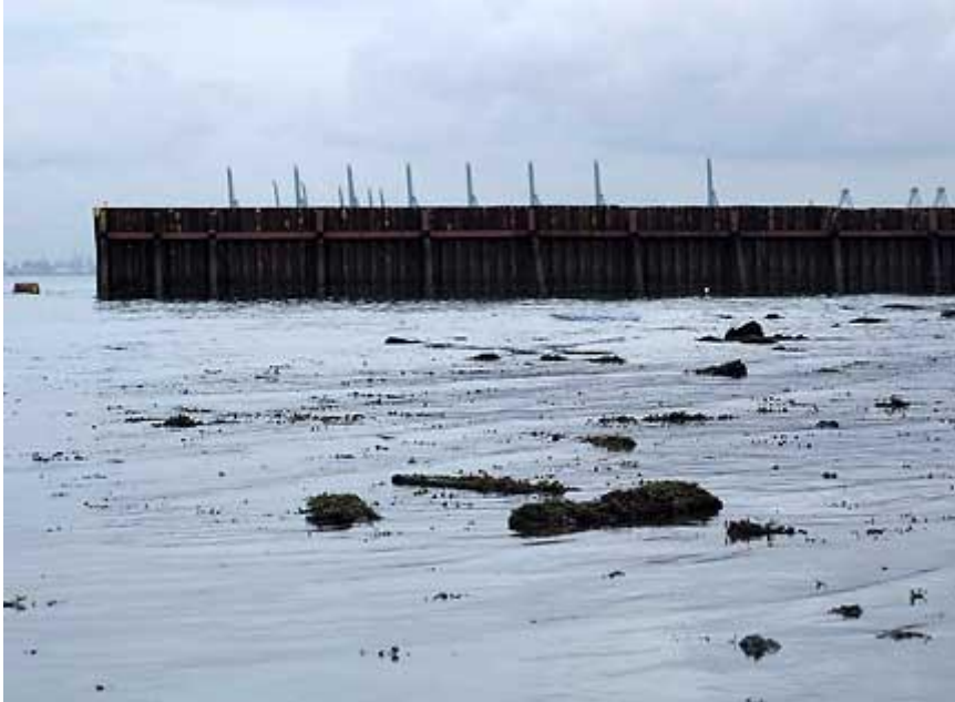
Figure 32: Typical example of a cofferdam in the shallow area
