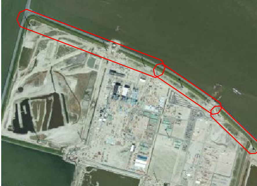
Figure 22: Eastern side of the Eemshaven
