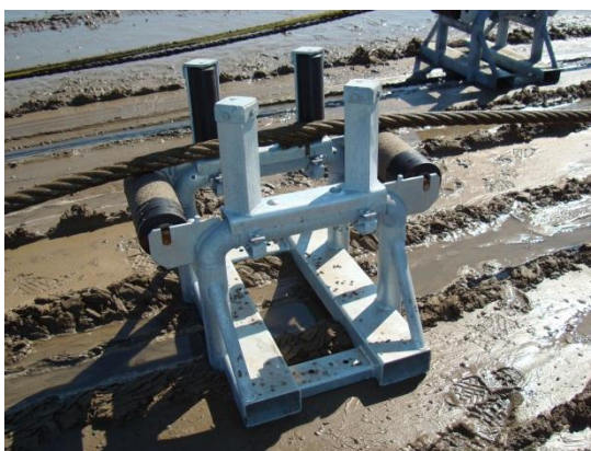
Figure 13: Detail of temporary roller
