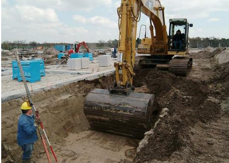
Figure 4: Trenching with a crane
