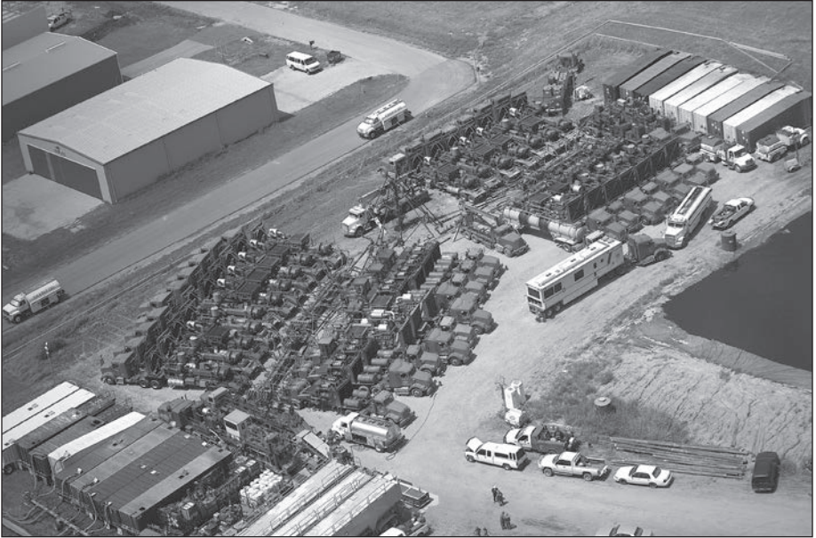
Fig. 3–5. Equipment assembled for a fracking job
