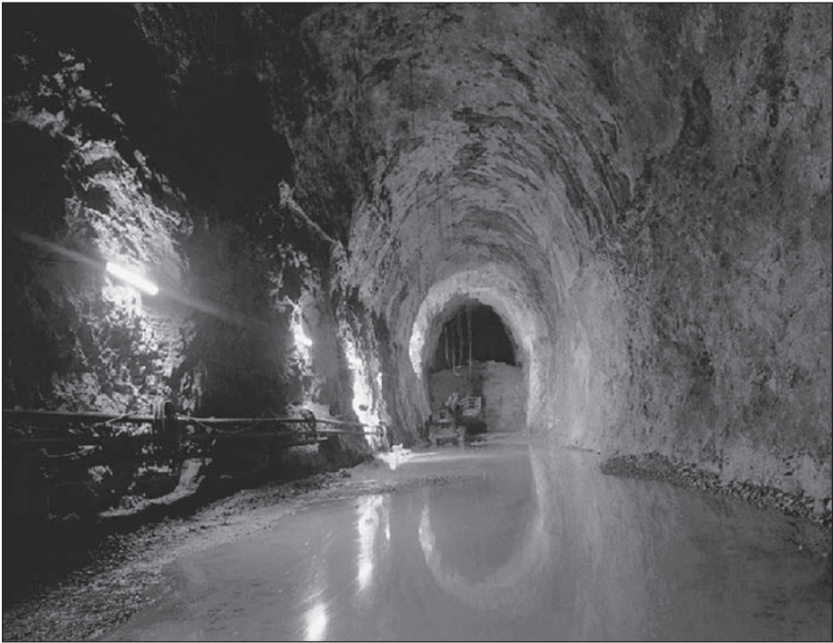
Fig. 7–13. Rock cavern ready to be filled (courtesy of Geostock US)
