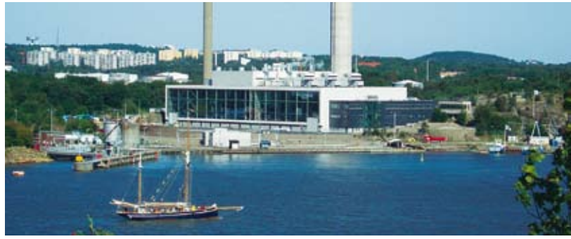
The combined-cycle cogeneration (district heating) plant of Göteborg Energi AB (Rya, Gothenburg) has a total efficiency of 94 %.
