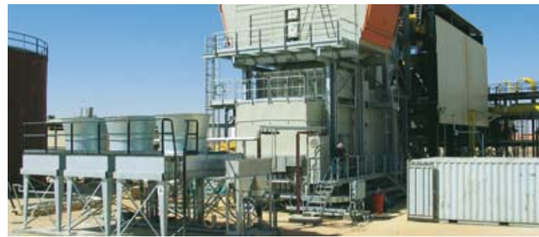
Compressor drive installation in Edjeleh, Algeria.
