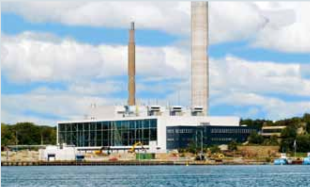
Göteborg Energi AB, Rya, Gothenburg: Three 45MW(e) SGT-800 gas turbines at the combined heat and power plant provide electricity and heating to the city of Gothenburg.
