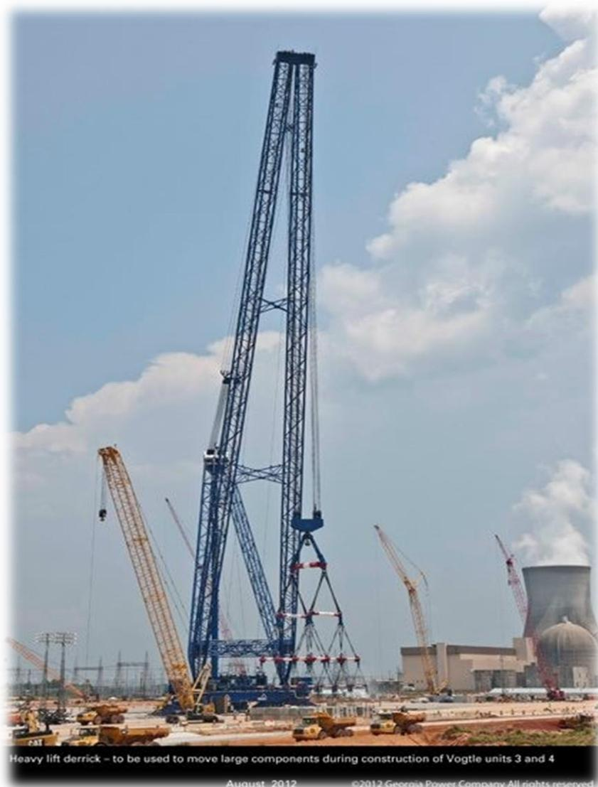
Bigge Crane & Rigging in the USA has its 125D AFRD, which it describes as the world's largest capacity crane at radius. Bigge gives the capacity of the ARFD as 7,500 US tons (6,800 tons) on 300 feet (91 m) of main boom and 4,000 tons (3,630 tons) with 560 feet (171 m) of main boom. Fixed jibs will be available in excess of 1,000 tons (907 tones) capacity and 200 feet (61 m) long, according to Pete Ashton, vice president of major projects.
