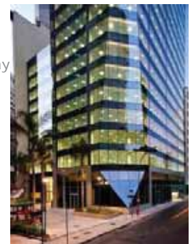
Rio Engineering Centre
