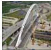
Calatrava road bridge
