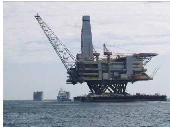
Sakhalin Island, Russia, integrated deck floatover installation
