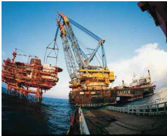
Saipem 7000 installing platform accommodation module
