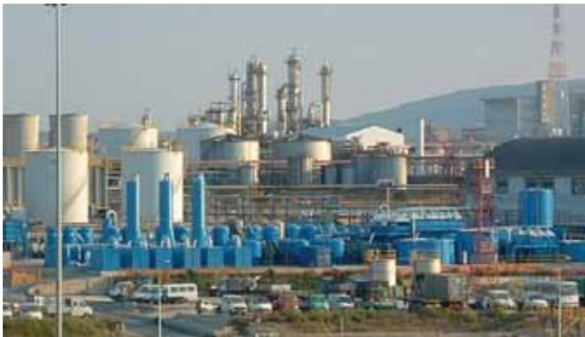
Groundwater Treatment Plant Porto Torres - Italy
