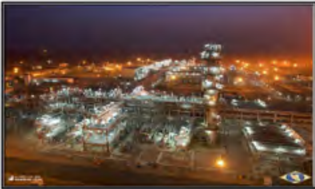
Darquain Oil Field Development
