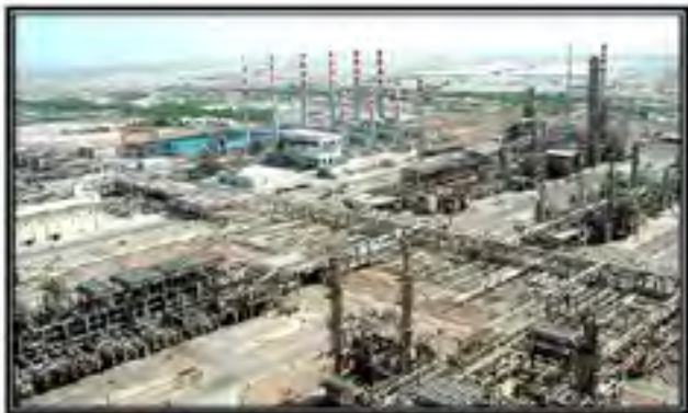
Bandar Abbas Oil Refinery
