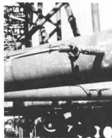
Fig. 19 Precious metal impressed-current anode on offshore platform prior to launching in the North Sea. Courtesy of W.H. Thomason, Conoco, Inc.
