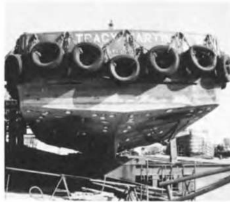
Fig. 16 Zinc anodes on the underside of a fishing boat
