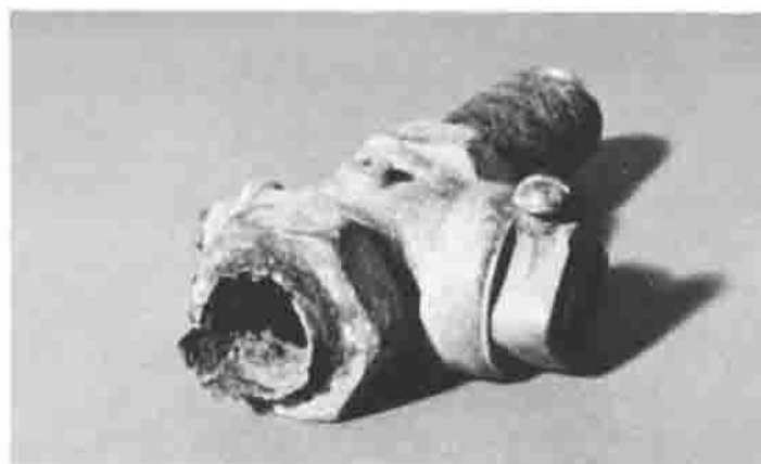
Fig. 13 Galvanic corrosion of steel pipe at brass fitting in humid marine atmosphere. Courtesy of R. Baboian, Texas Instruments, Inc.
