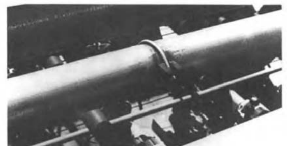
Fig. 2 External clamping used to stop leaks
