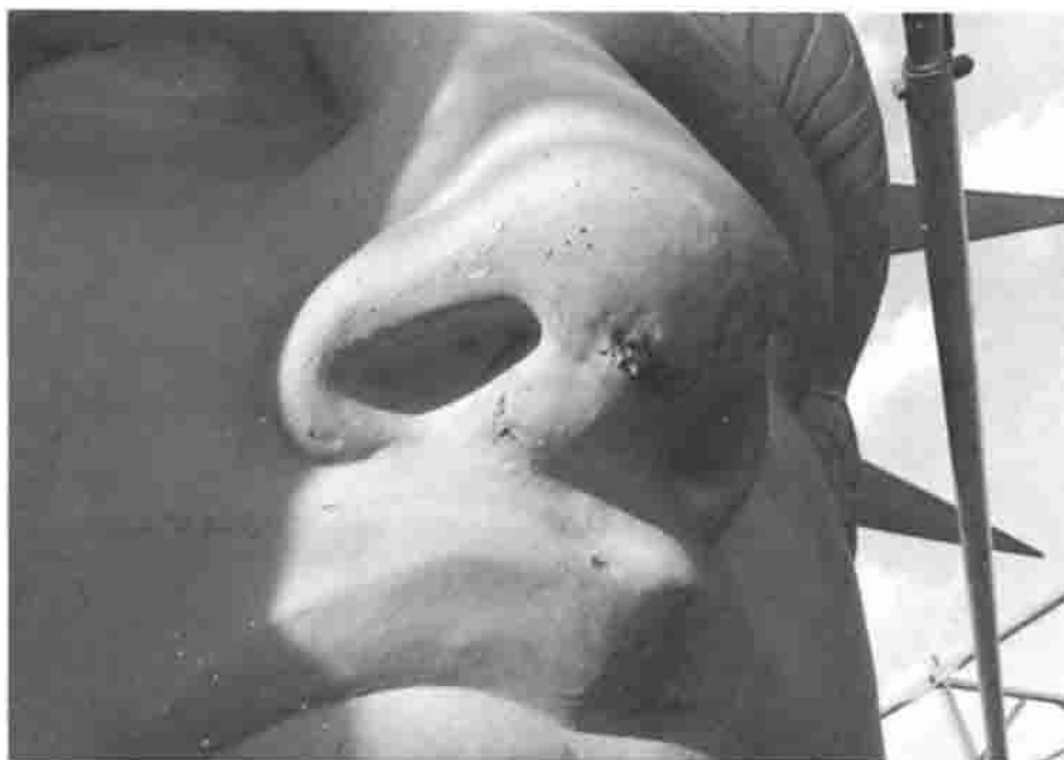
Fig. 11 Moisture that collected on the inside of the Statue of Liberty caused galvanic corrosion of the iron armature in contact with the copper skin. The copper skin on the nose was ruptured due to mechanical forces of the resulting corrosion products. Courtesy of R. Baboian, Texas Instruments, Inc.
