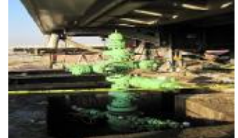
MJ-E22a-01 The first newly drilled & completed SIPD well
