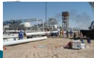
DS1 - Bypass line installation and welding
