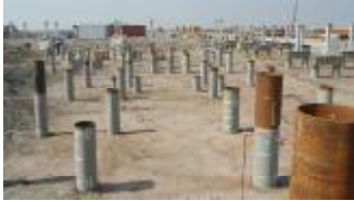
Piling for Train 1 skids
