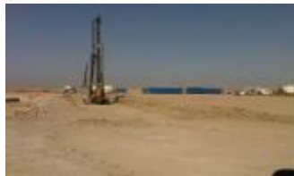
Pile driving unit on location at MJ-E22 drilling pad
