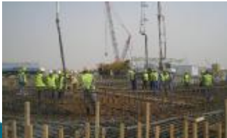
Produced water tank foundation
