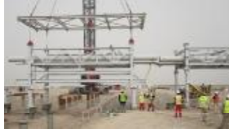
Piperack Module 21 lifted by 600T crane and fitted with Module 23
