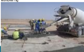
Pouring concrete base for cellars at MJ-E20 drilling pad
