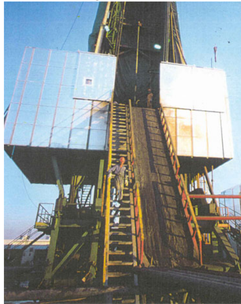
Rig floor area
