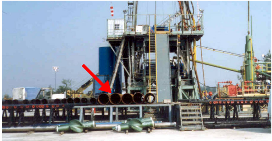
Pipe rack: Casings
