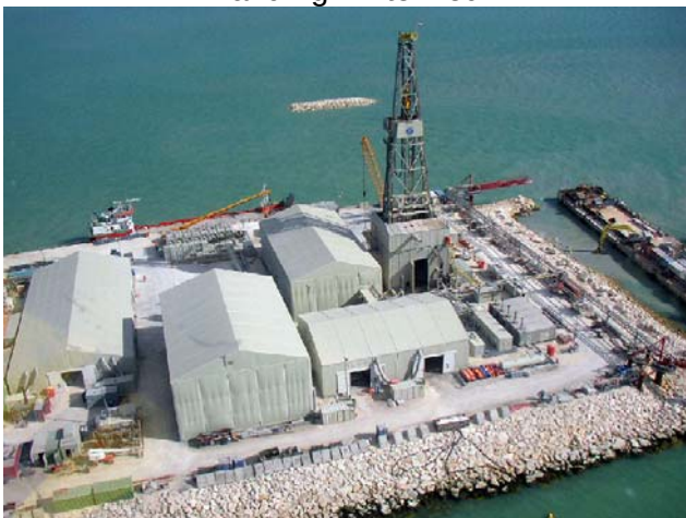
Land rig winterized
