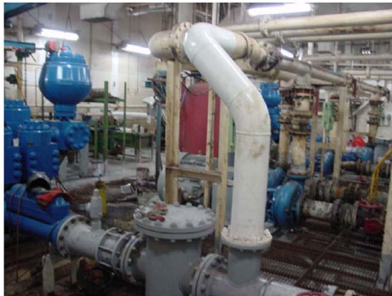
- Pulsation dampener on discharge line
