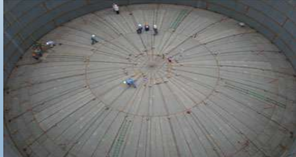
直径60米罐顶铝网壳 60m Diameter Triangular Aluminum Dome of Tank
