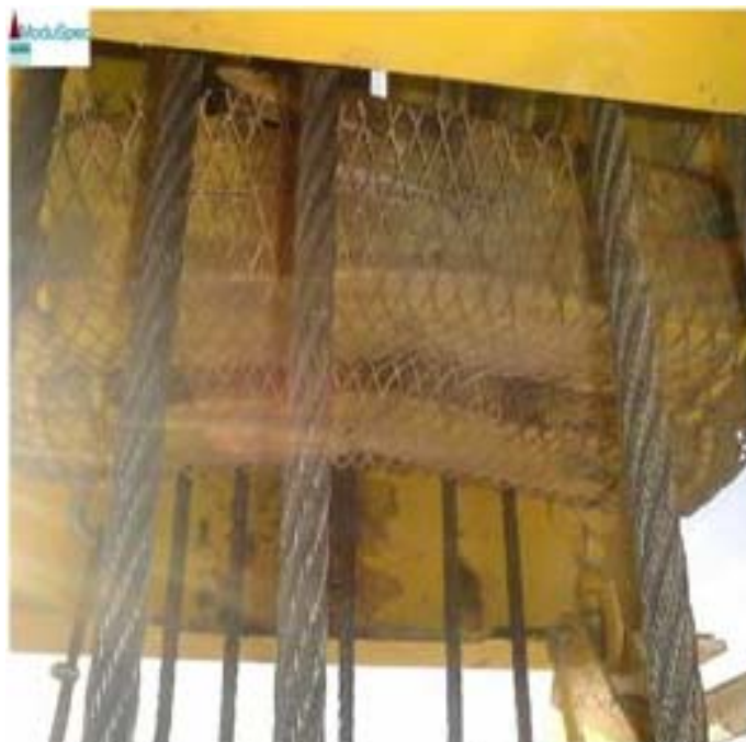
Figure 27 - This is what is meant by substantial wire mesh.
