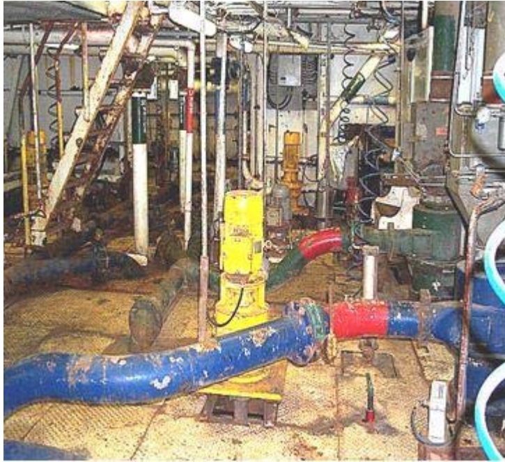
Figure 22 - Mud-mixing equipment layout.
