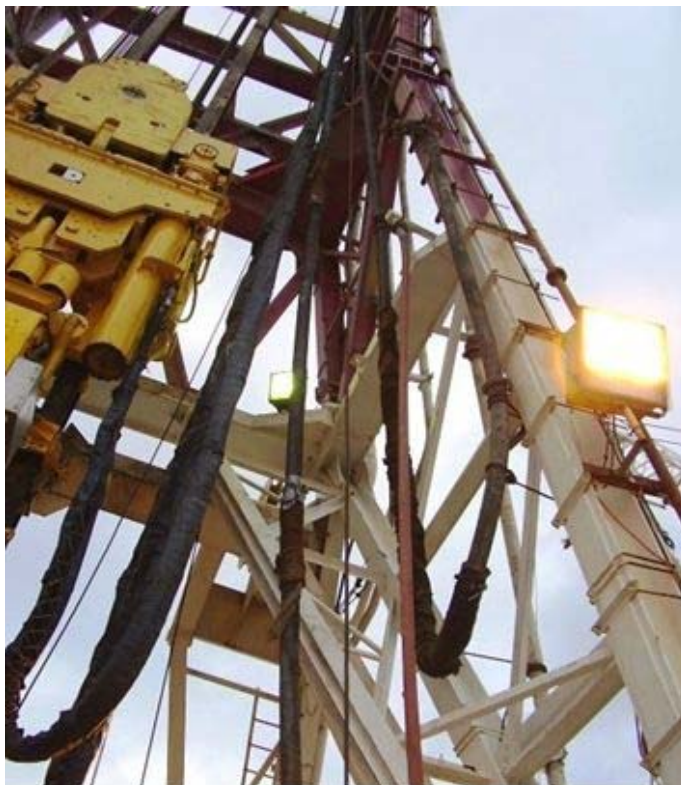
Figure 17 - Spare hose in derrick.
