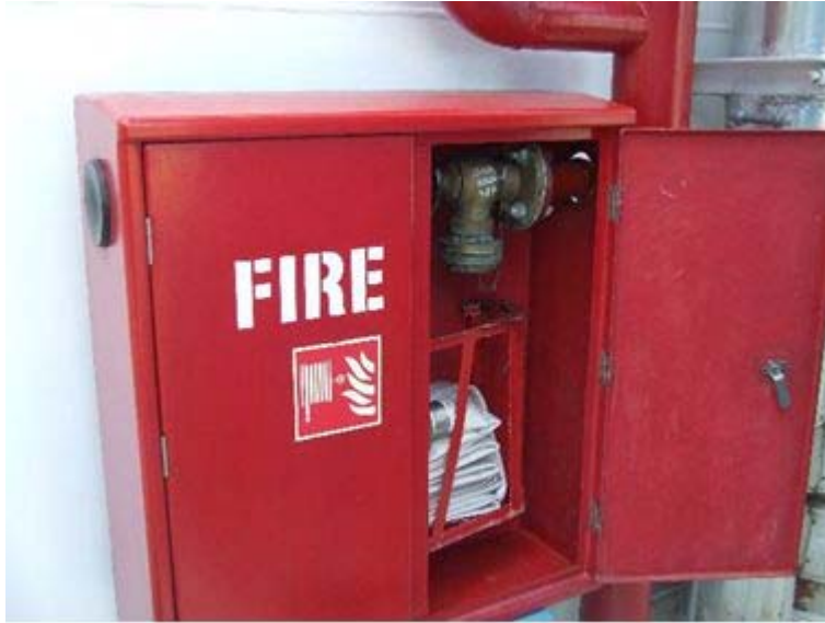
Figure 2 - Typical fire hydrant
