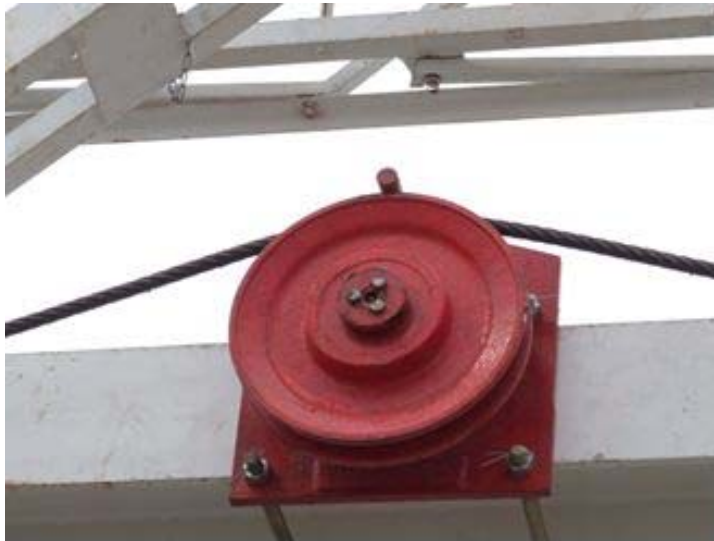
Figure 37 - New raising-line sheave.
