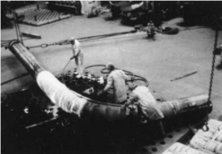
FIGURE A6.12 Hot bending on a table. ( Pullman Power Products Corporation )
