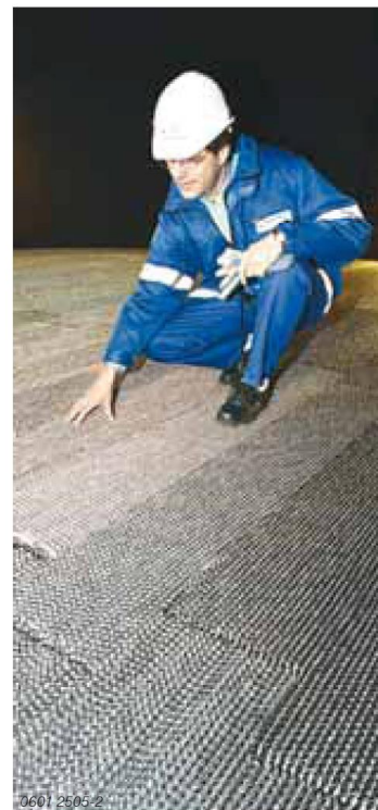
0661 2505-2 Inspecting packings after installation
