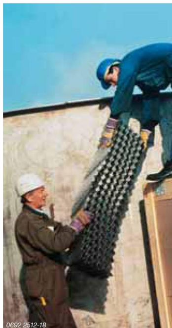
0692 2512-18 Revamping of a vacuum column with Mellapak
