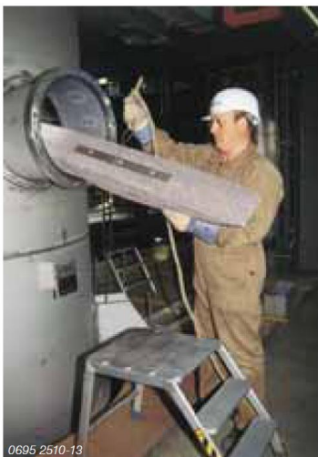
0695 2510-13 Installation of packing
