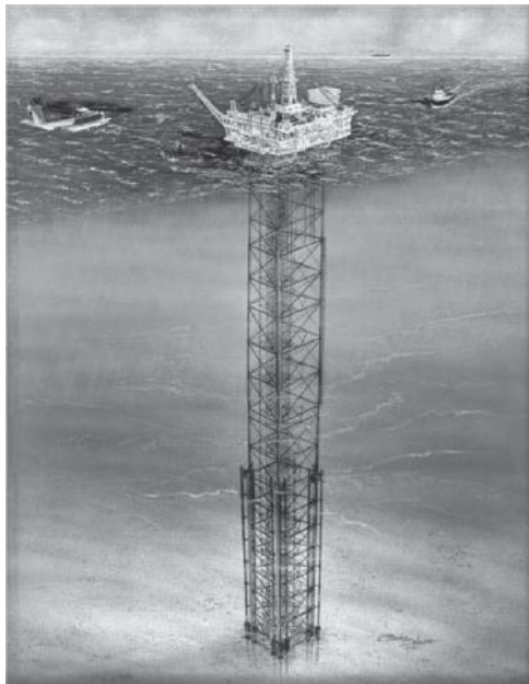
FIGURE 1.24 Petronius compliant piled tower platform. (From Petronius Compliant Tower. Courtesy of offshore-technology.com . With permission.)
