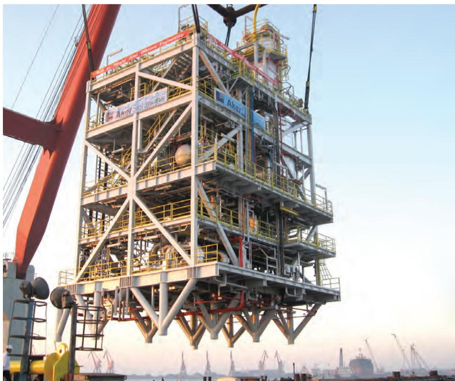
Figure 4.8 – Processing equipment ready for installation to improve oil and gas production. Courtesy: AkerSolutions
