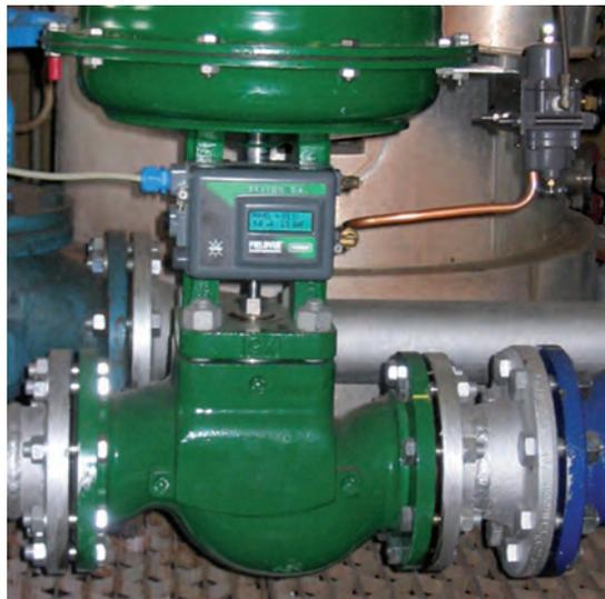
Figure 7.5 – Globe control valve with pneumatic actuator and smart positioned.
